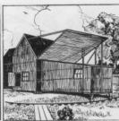
In the Edison laboratory yard at Orange, N. J. the first of all motion picture studios was built. It was a wooden, barnilke structure with a roof that could be resized and lowered. It revolved on a circular track and was swung with the sun. Black roofing paper covered the bindle and outside. It was called the "Black Maria."
